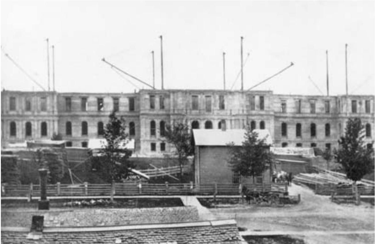
The Capitol under construction, ca. 1875. Derricks rise above the walls, which have been completed to the second story.
